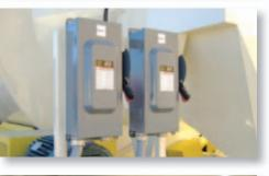
Enables isolation of each motor for maintenance and reduces expensive field wiring
